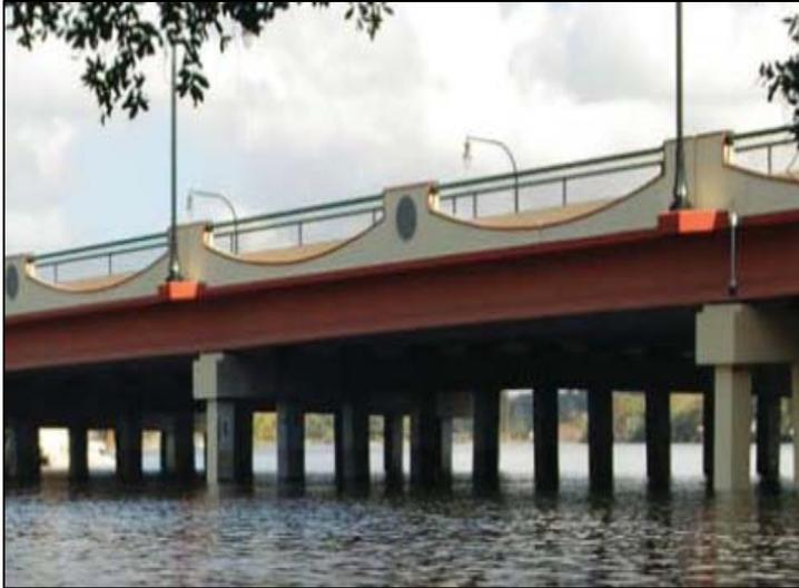
As featured in the spring 2009 issue of ***ASPIRE Magazine***, "...The 40<sup>th</sup> Street Bridge in Tampa, Fla., features a single post-tensioned concrete span with special aesthetic treatments created by local high-school art students. They learned the basics of conceptual design, and contest winners had their designs' ideas, colors, and shapes incorporated into the formal aesthetic plan.
